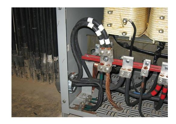
An assured equipment grounding conductor program verifies all the grounding points inside all equipment.
