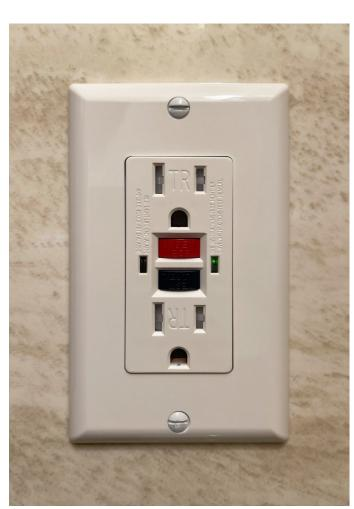
GFCI receptacle with red button for Reset and black button for Test
