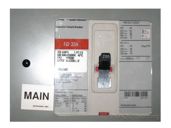
The interrupting rating of a device cannot be less than the available fault current at that location.
