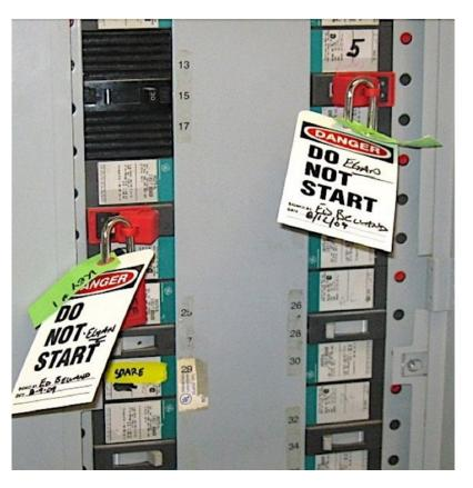
Conductors and circuit parts locked and tagged in the disconnected position are part of securing an electrically safe work condition.
