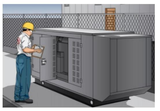
Once equipment has been successfully field evaluated, a field label is applied. In many cases, a field label is accepted by the NFPA in lieu of a regular product listing.
