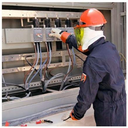
Protective clothing must protect workers from both shock and arc flash hazards.
