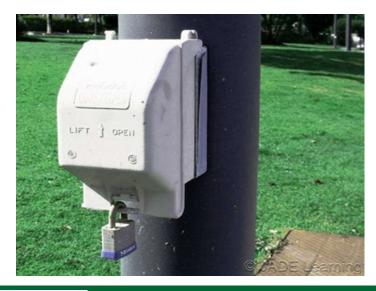
An outlet box hood is a housing shield intended to fit over a faceplate for flush-mounted wiring devices, or an integral component of an outlet box or of a faceplate for flush-mounted wiring devices.
