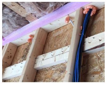
Cables installed parallel to wood framing must be installed at least 1.25 inches from the nearest edge of the framing member in accordance with 300.4(D).
