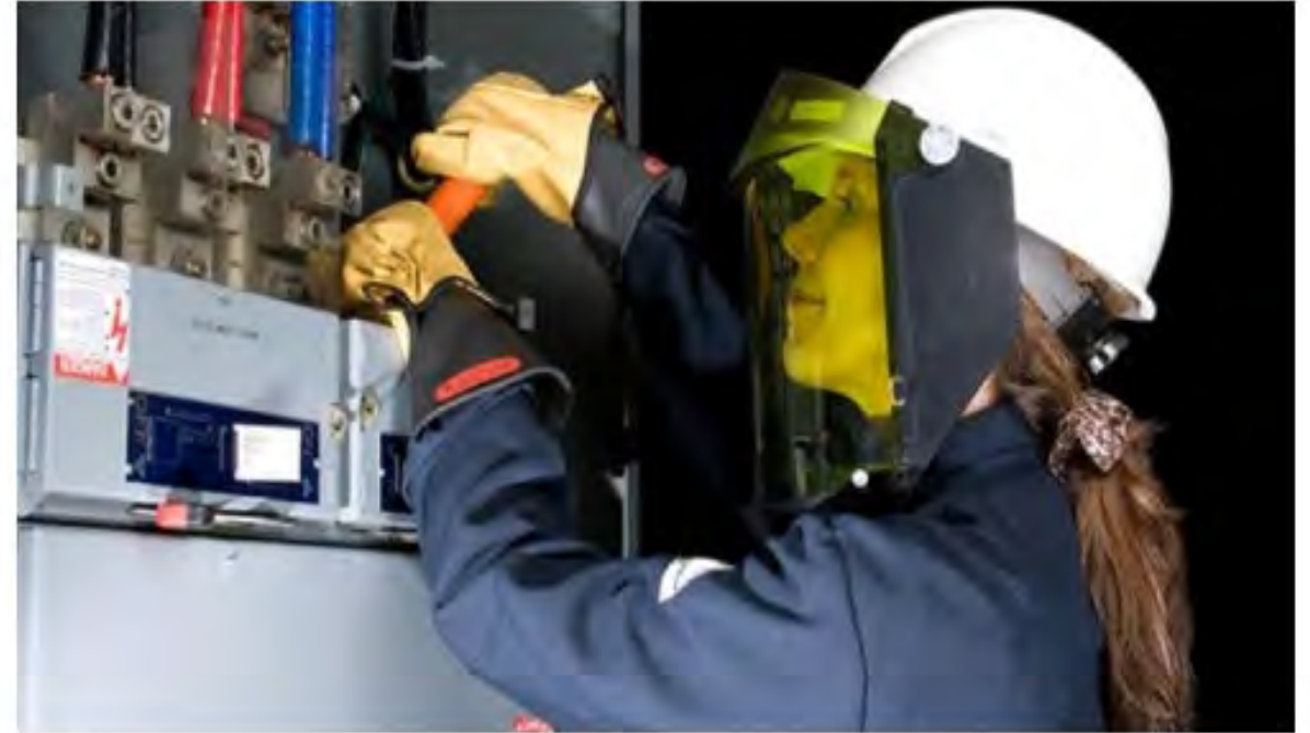
Personal Protective Equipment (PPE) protects personnel from electrical hazards.
