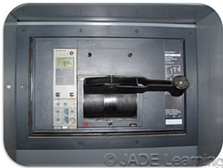
Ground-fault protection is required on large services.
