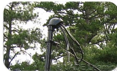
Service heads and goosenecks must be located above the point of connection of the service-drop conductors.
