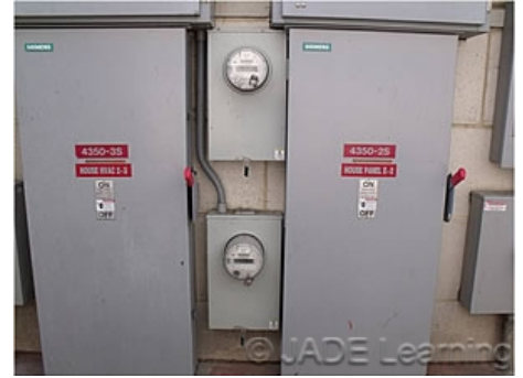
Service disconnects must be grouped in one location and marked to show the load served.
