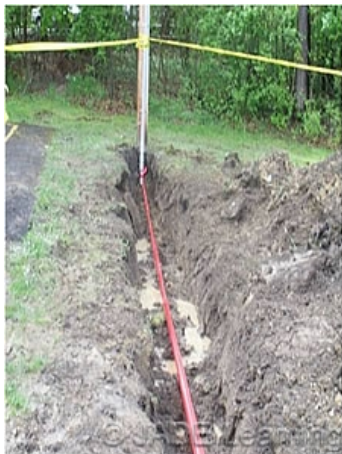
Underground service conductors must be protected from physical damage. Cover requirements are determined by Table 300.5.
