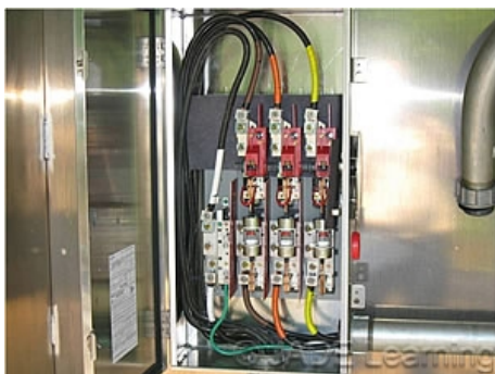
Service entrance conductors are sized according to Article 220 for the calculated load.
