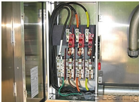
The overcurrent device must be part of the service disconnecting means or immediately adjacent to it.
