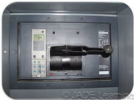
Ground-fault protection is required on large services.
