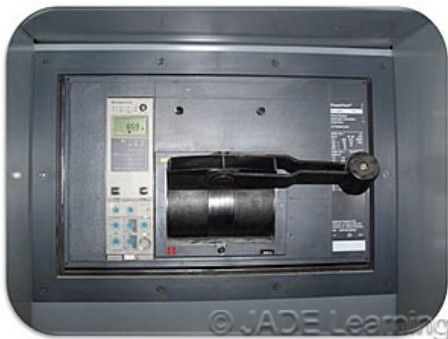
Ground-fault protection may be required for some services.
