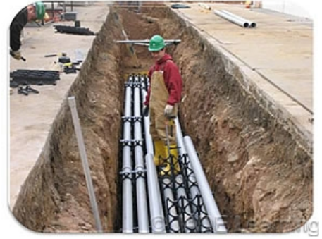
Underground service-entrance conductors are installed between the terminals of the service equipment and the point of connection to the service lateral or underground service conductors.
