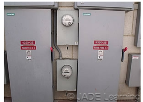
Service disconnects must be grouped in one location and marked to show the load served.
