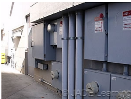
Service Equipment includes the circuit breakers and fused switches to disconnect all the ungrounded conductors from the service-entrance conductors.
