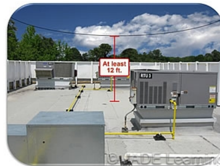
A clearance of 12 ft. is required over flat roofs subject to pedestrian traffic when the voltage to ground is over 150 volts but not over 300 volts.
