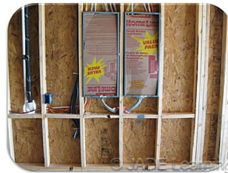
The service disconnect(s) must be installed at a readily accessible location nearest the point of entrance of the service conductors.
