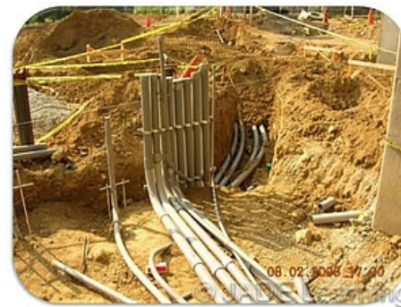
RMC, IMC, EMT, RNC, Type MC Cable, FMC or LFMC not over 6 ft. long, & LFNC are permitted wiring methods for service entrance conductors.
