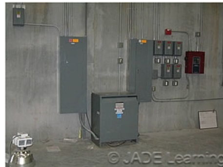
Overcurrent protection on the secondary side of a transformer can be omitted if the tap conductor on the secondary side of the transformer meets all the conditions in this section.
