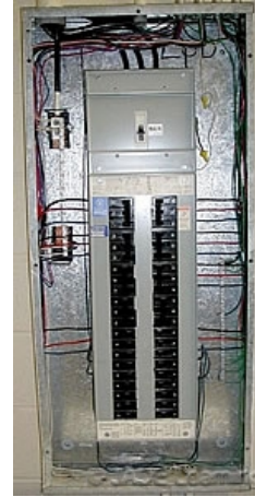
The rating of OC protection for a panelboard cannot be greater than the rating of the panelboard busbars.
