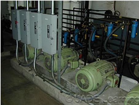
Branch-circuit and short-circuit protection for a single motor is selected from Table 430.52, based on the full load current of the motor.
