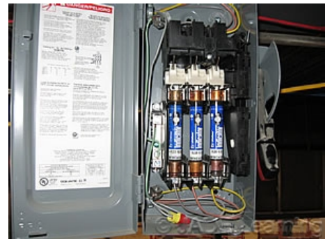
Continuous loads are protected at no less than 125% of the calculated current.
