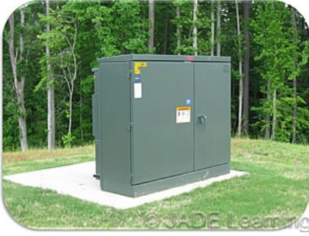
Overcurrent protection for transformers with primaries or secondaries rated over 1000 volts is selected from Table 450.3(A).
