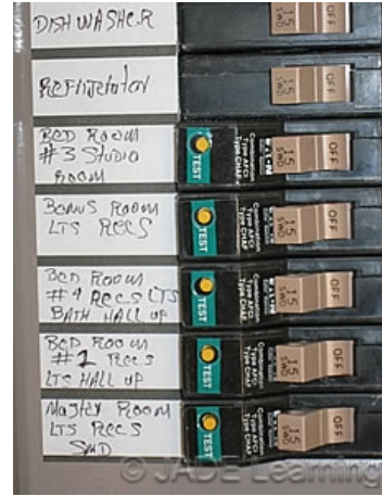
Combination type arc-fault circuit-interrupter protection is required in those locations in a dwelling that require arc-fault protection.
