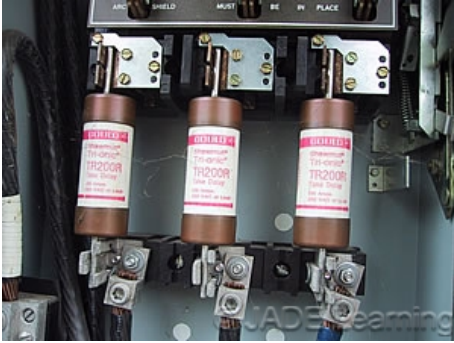
A motor feeder that supplies more than a single motor is protected according to the requirements in Code section 430.62.
