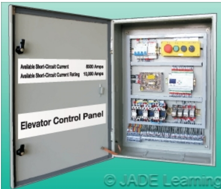
Elevator control panels must be marked with a short-circuit current rating. The short-circuit current rating of the equipment must be greater than the available short-circuit current.
