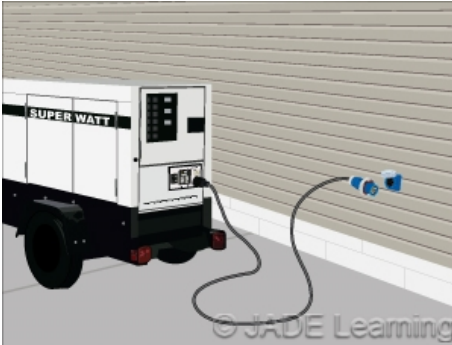
Power inlets rated 100 amperes or more that are used with outdoor portable generators must be listed for the intended use.
