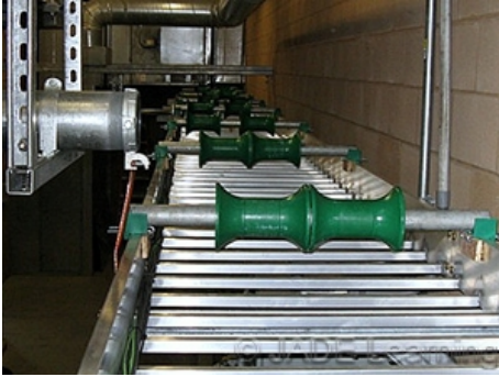
The continuity of equipment grounding is maintained from this raceway to cable tray.
