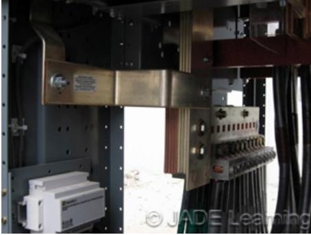
Equipment bonding conductors are installed with each parallel run of ungrounded conductors.
