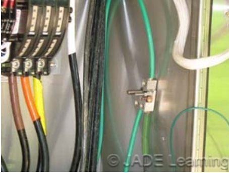
The re-identification of conductors in multiconductor cables as equipment grounding conductors is required at every device, junction box, distribution panel, or other location where the wiring is accessible.
