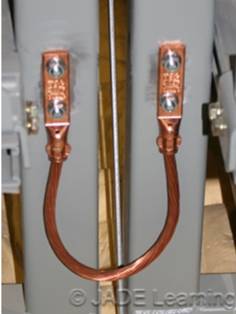
The ground-fault path between these two metal racks is ensured with a bonding jumper.
