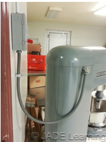
This fixed bakery dough mixer has metal parts that could become energized and must be properly grounded.
