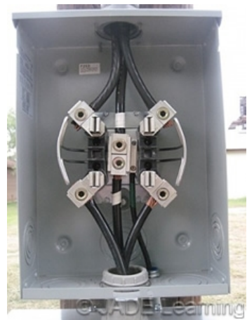
250.142 permits the use of the grounded service conductor for grounding equipment on the supply side of the service disconnecting means.
