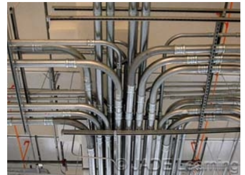
This installation utilizes EMT and couplings made up wrench-tight to maintain effective ground fault path.
