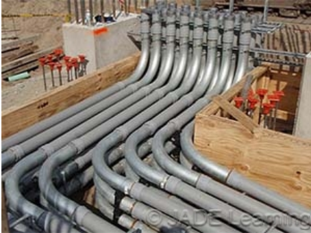
A full sized equipment grounding conductor is required in each raceway when paralleled conductors are installed in multiple raceways.
