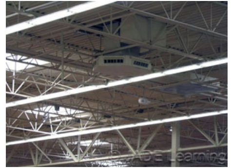
Luminaires and associated equipment are required to be connected to one of the 14 types of equipment grounding conductors that are listed in 250.118 and sized as required by 250.122.
