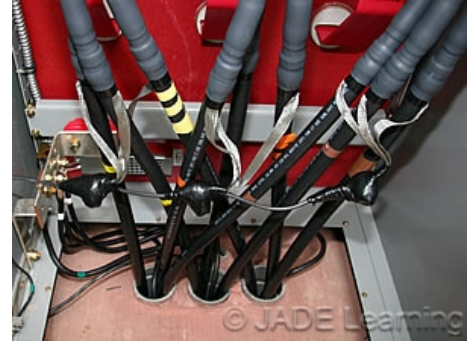
Equipment grounding conductors are required for medium voltage circuits.
