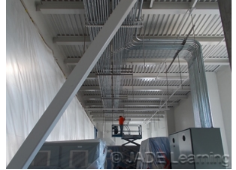
This conduit run maintains a conductive path connecting the non-current-carrying metal parts to the grounding electrode conductor.
