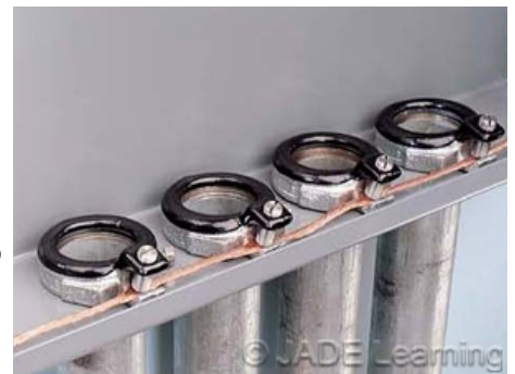
Pre-punched knockouts are considered impaired connections and will require bonding bushings or jumpers to maintain fault-current path.
