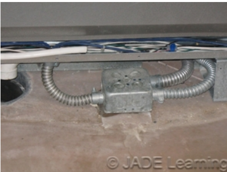
Flexible metal conduit is permitted as an equipment grounding conductor with 20 amperes of overcurrent protection or less.
