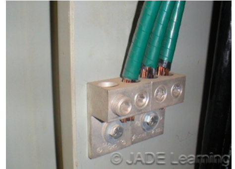
Conductors larger than No. 6 AWG are not required to have a continuous green outer finish.
