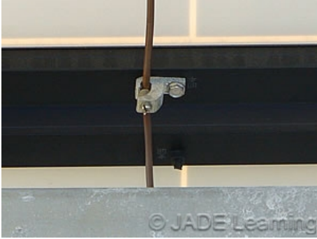
Non-current-carrying metal parts of a PV system must be bonded together and connected to an equipment grounding conductor.
