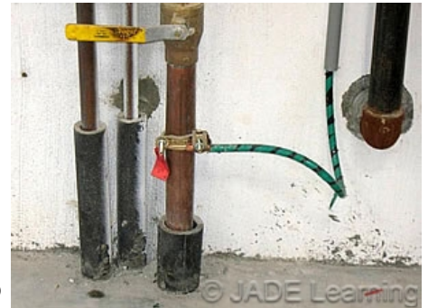
The first 5 feet of metal water pipe above ground is permitted to extend the connection to the grounding electrode (water pipe).
