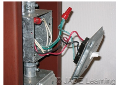
Snap switches, dimmers, and similar control devices must be grounded and provide a way to ensure continuity with metal faceplates.
