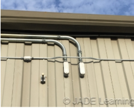
Raceways entering a building from outside must be sealed.
